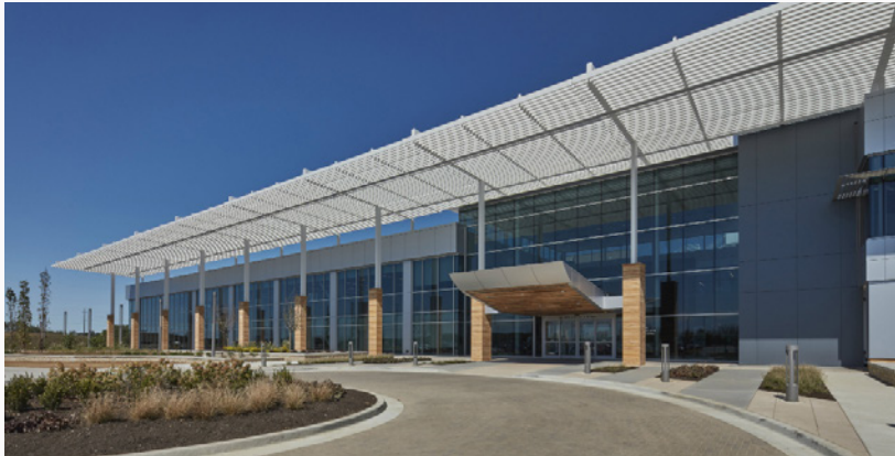
The Toyota Production Engineering and Manufacturing Center in Georgetown, Kentucky, was awarded Platinum LEED® in April 2019.
